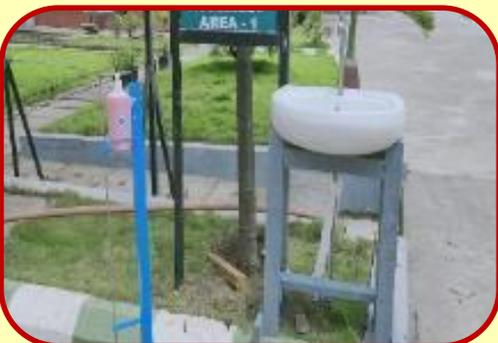
Touch free (Foot operated) hand washing basins installed at various places.
